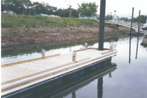
Wheelchair Border on floating dock
