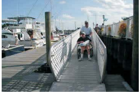
ADA Gangway and railing
