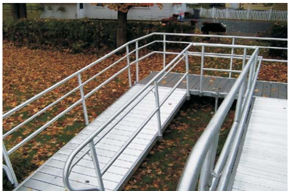
ADA Residential ramp
