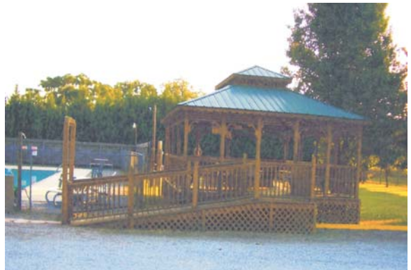
Wheelchair Ramp w/ landing and turn
